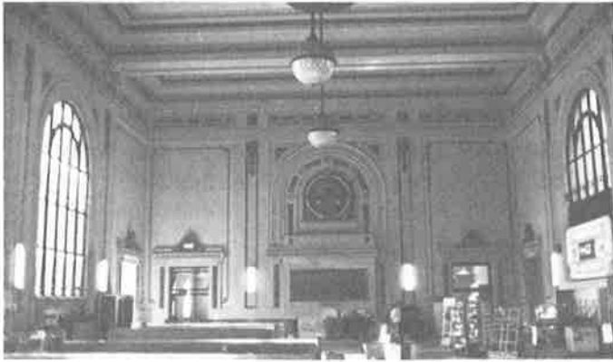
Interior of 16th Street depot, built 1912.
