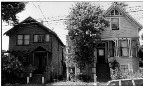
BROOK STREET: auto shop, top, and two homes, bottom, to be removed.
