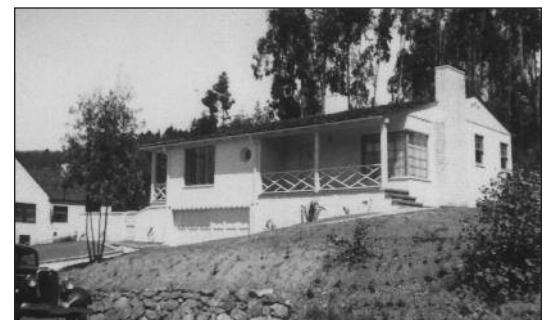
TIKI ROOM at top: paneling, knotty pine, mirrors and original tropical-themed wallpaper. Above: Duncan Way exterior with then-modern car.
