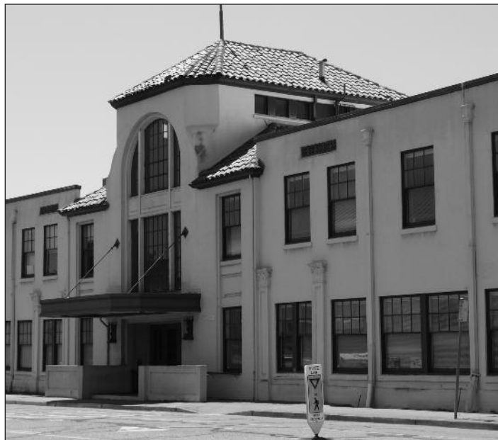
OAKLAND AIRPORT'S NORTH FIELD.
