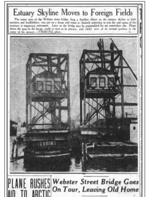
NEWSPAPER REPORT on the bridge's removal in pieces.
