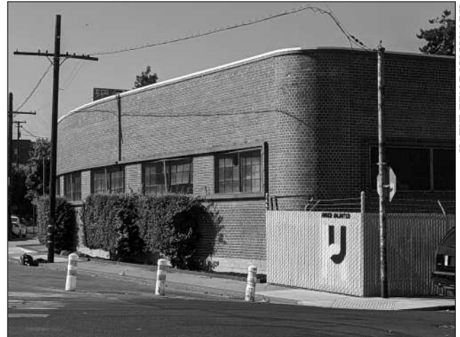
A CURVING WALL at 5303 Adeline St. signals mid-century allure.
