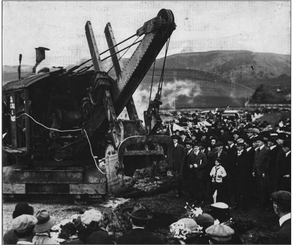
BREAKING GROUND for the new Chevrolet plant in East Oakland, 1915.
