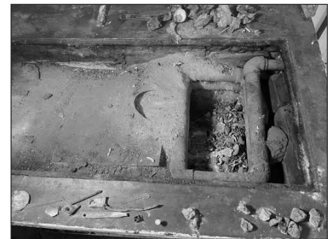
PERHAPS LUCKILY , the old stove hadn't been cleaned before sealing it up, so it provided intriguing clues. At top right, the pipe is evidence that this kitchen stove at some point furnished heated water upstairs.
