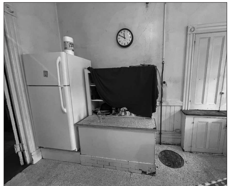
THE COUNTER next to the fridge hid the old coal range.
