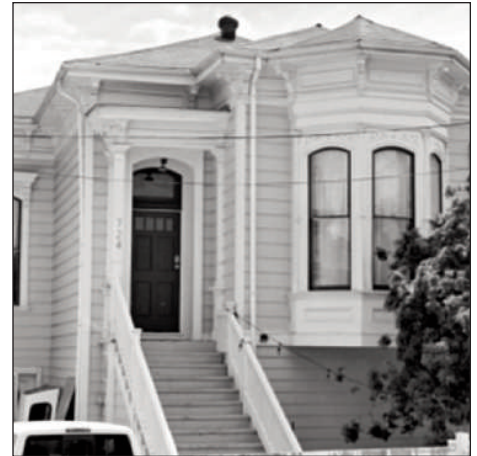
CITY OF OAKLAND
