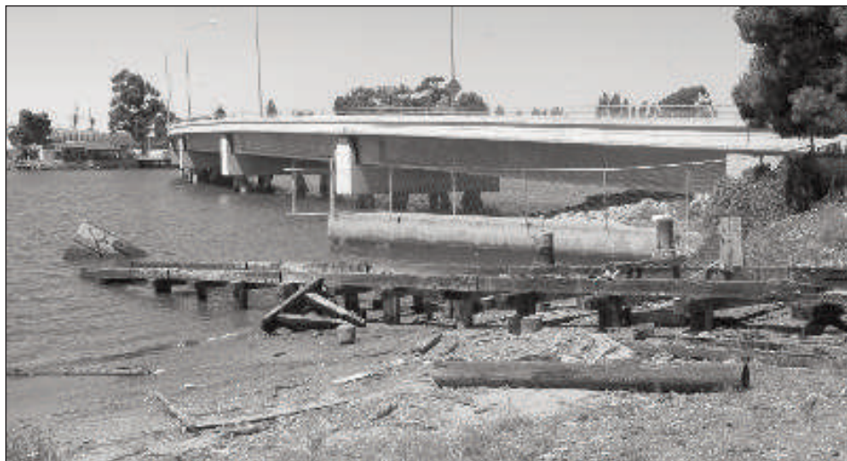
THE CRYER SLIPWAY that once permitted ships to enter the water. This photo was taken in 2013.
