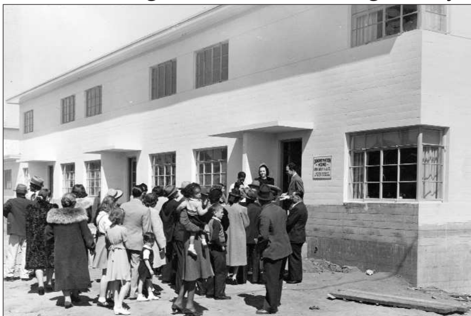
PEOPLE WAIT to see a newly-constructed model home at Peralta Villa.
