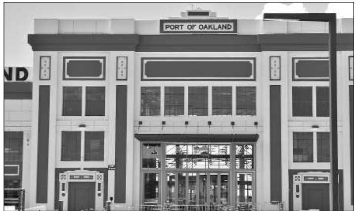
HEADHOUSE AND FIRST 120 FEET of 9th Avenue Terminal still stand; exposed trusses and a partial wall serve to indicate its former extent. Interpretive plaques such as the one below explain the history.
