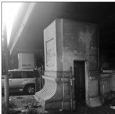
POSEY LOST ITS PETALS: To accommodate the freeway, pillars were cut off.
