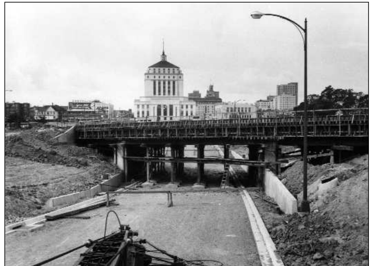
WHAT GOES UP must come down: the viaduct under construction.
