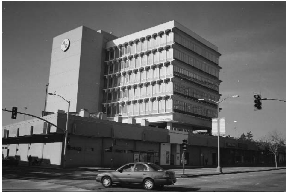
ONCE CONSIDERED GROUNDBREAKING , the M/B Center has seen better days . . . but won't have any at all soon. Demolition is underway.
