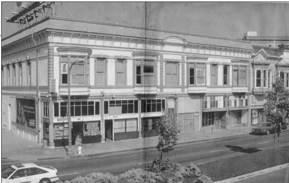
THE HISTORIC HANIFIN BLOCK on San Pablo Avenue
