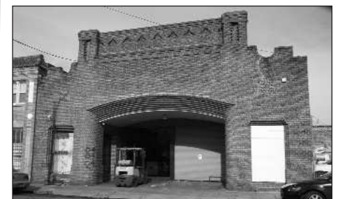
THE DOWNTOWN PLAN includes the historic 25th Street Garage District area, home to Art Murmur, with early auto-oriented buildings such as this one, constructed 1929–30.
