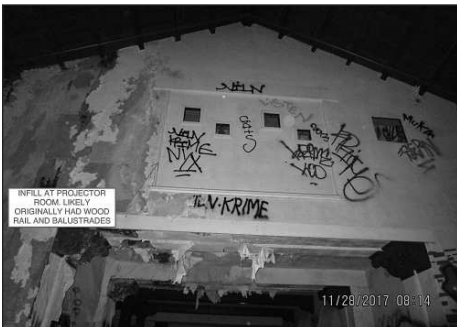
AN ORCHESTRA BALUSTRADE was likely here before the Projection Room was installed.
