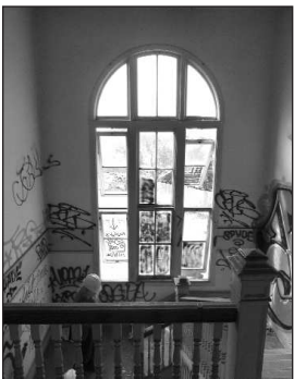
STAIRWELL in the Ethel Moore Building.
