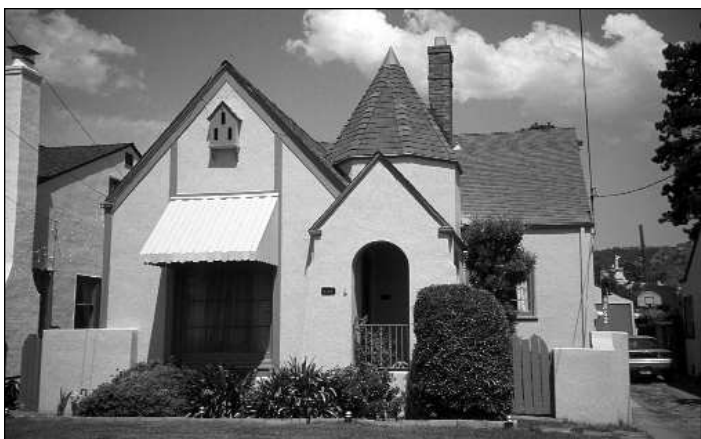
AN ORNAMENTAL TRIPLEX BIRDHOUSE adorns this home in the charming Picardy neighborhood.
