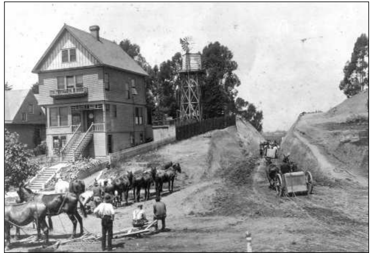
EARLY CONSTRUCTION WORK on Piedmont Avenue.
